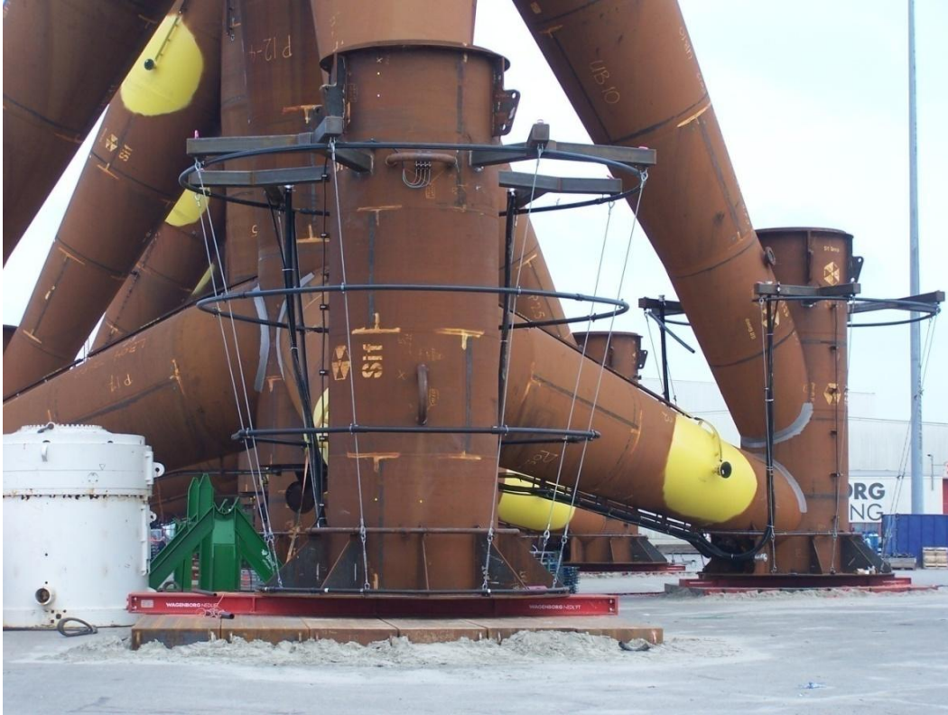
AV09 in testfield alpha ventus with pre-installed lower part of tube system, designed by MENCK
